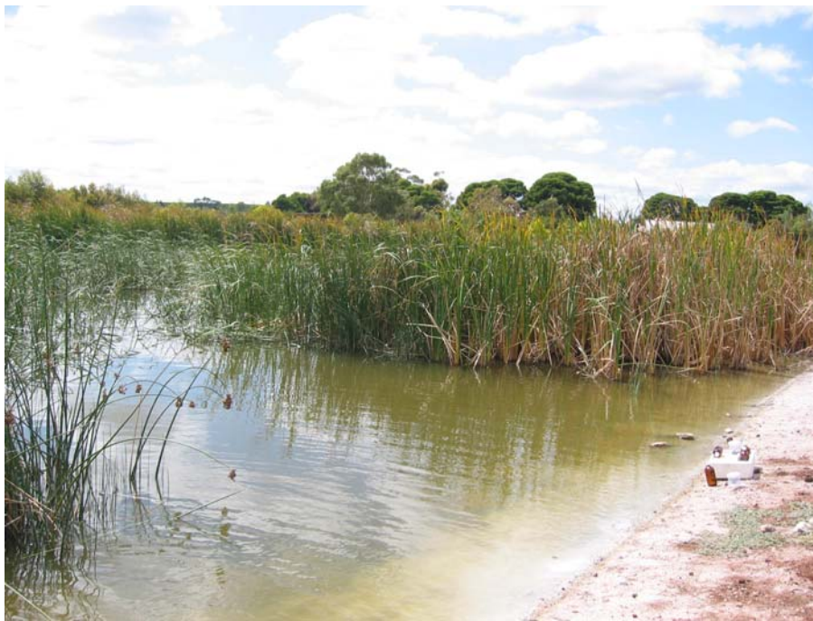
Figure 5.2 Dam receiving winery wastewater after passing it through a series of four cells.
